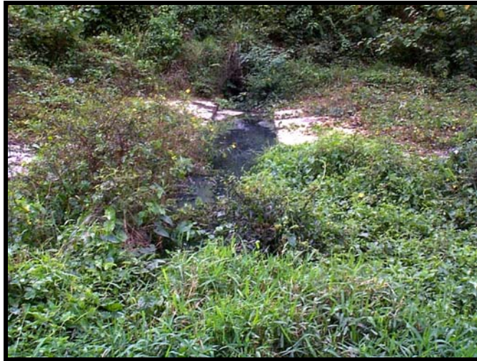
Photo 1: View of 24 inches drainpipe under Highway PR-30.
