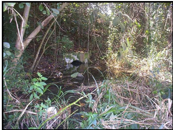
Photo 2 & Photo 3: View of 24 inches drain pipes that empty onto wetland area located in the southern part of the parcel.
